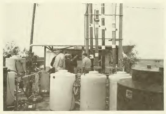
The anaerobic-bacterial process of removing selenium from drainage water was tested in this small plant near Mendota in 1986 and 1987.
