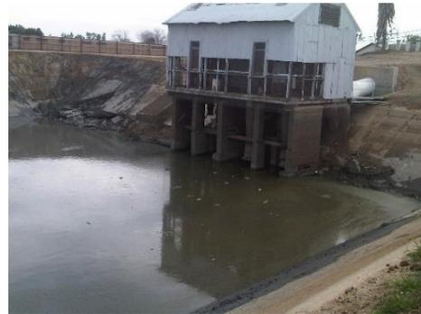
**Existing District Main Canal Pump Station – Note the Buckling Support Pillars**
